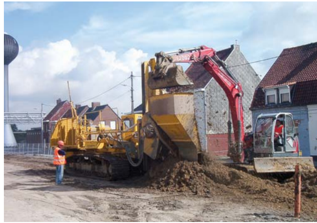
Installation of the drains
