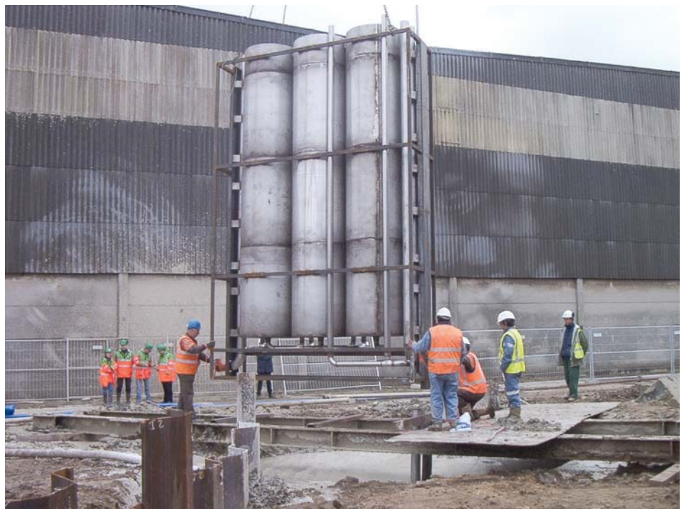
Placing of the filter gate
