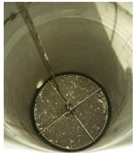
View of installed treating product
